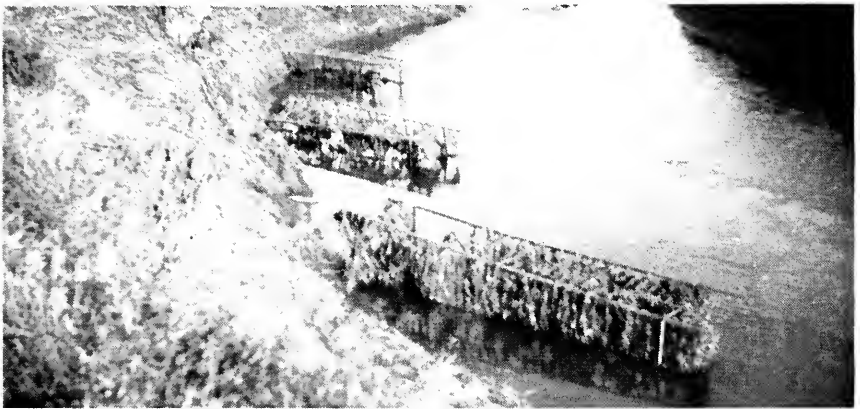
Fig. 11—Typical installation of fascine boxes.
